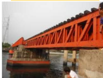
Steel red bridge
